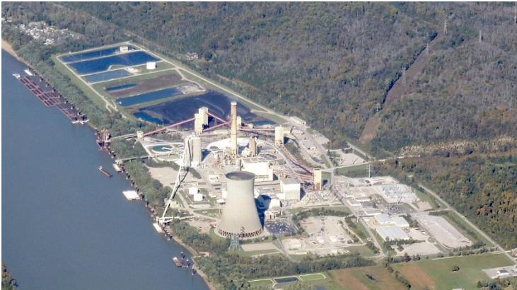
Figure 9: Integrated Ash Management Facility [11]
