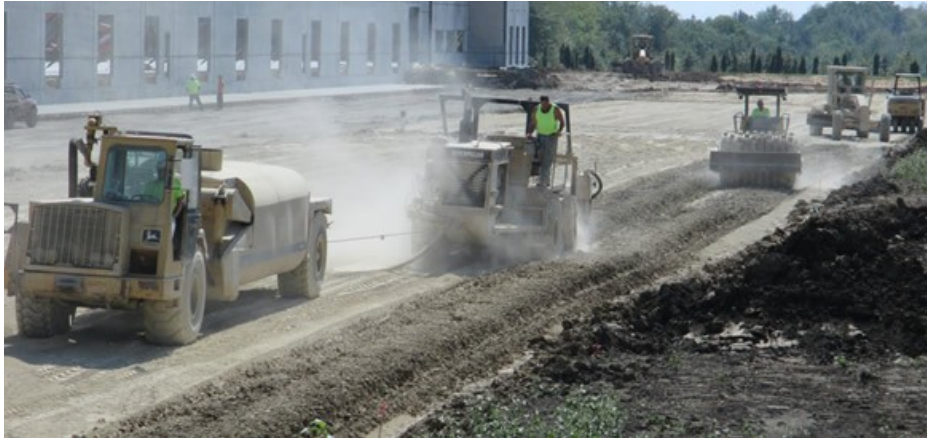
Figure 15: Utilization of Ash in Improving Soil Quality [76]
